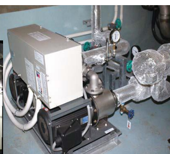
(iii) Boiler water supply pump
