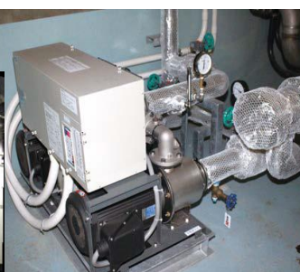
(iii) Boiler water supply pump
